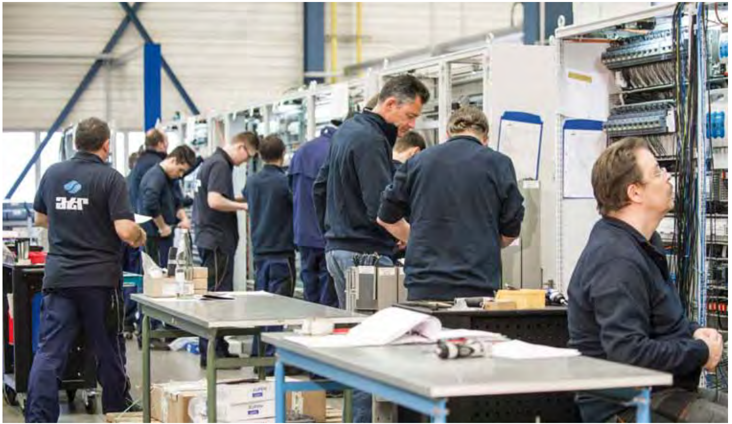
Switch cabinet assembly, ATR
